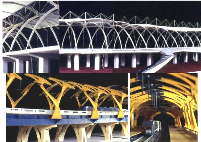
**Figure 13:** Selected designs for MRT stations. Aside from considering issues of structure, construction, and economy, the forms are also refined for visual elegance and identity from both the exterior and interior. These designs and details are by (top) Reyes et al, and (bottom) Tambis et al.
