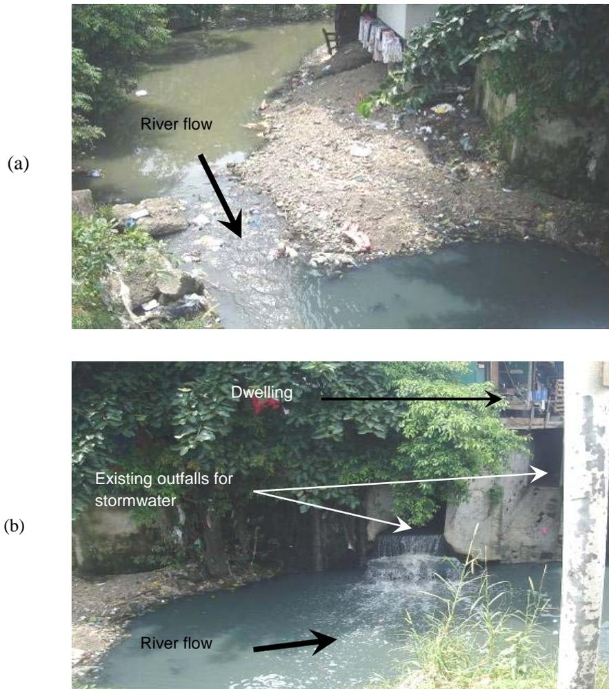
**Fig. 7** Conditions at the river outfall of municipal drainage system: (a) looking downstream; (b) view upstream
