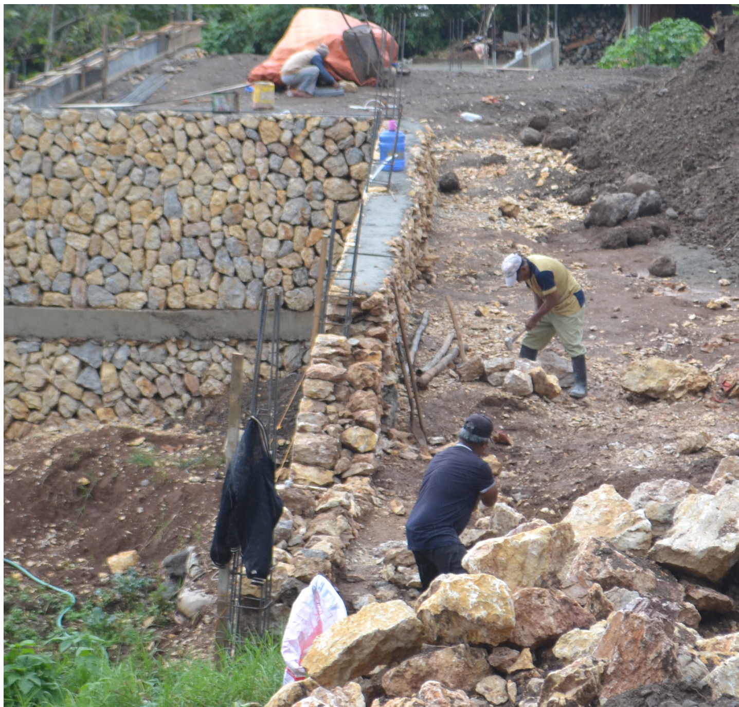
Kabite or riprap stabilizes the land (Photo by Dale Mercurio)
