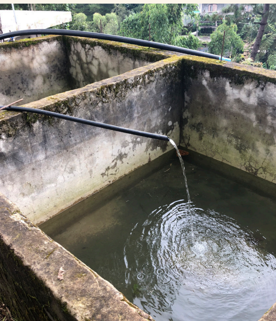
Pumped spring water to the household reservoir through a hose
