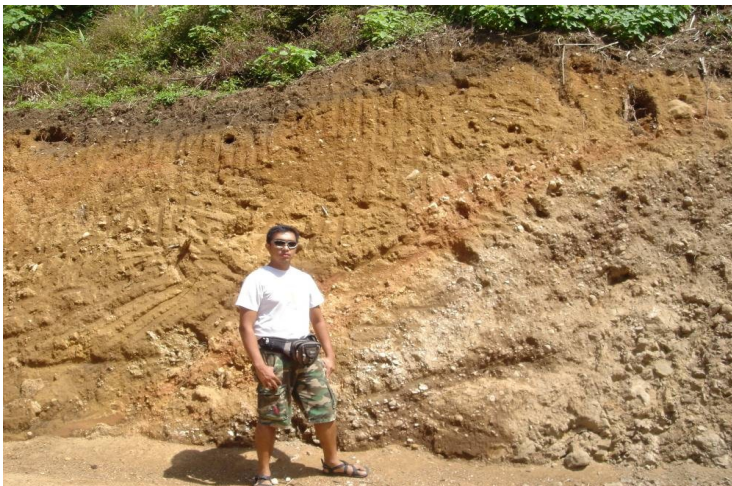
Figure 3: Example of a road cut at Mount Kabuyao, Sitio Poyopoy, Brgy. Taloy Sur, Tuba, Benguet. Notice thin topsoil interspersed with 20-30cm Layer A, 20-50cm Layer B is regolith. 300-500cm Layer C is mother rock (Photo taken by author April 2012)
