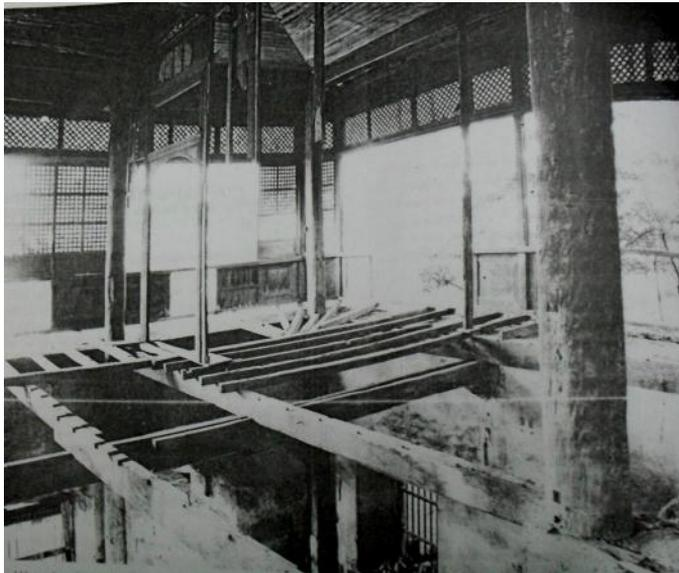
**Figure 25:** Photo of a framing structure of a bahay na bato in Taal, Batangas. Similar framing system may have been used in Structure A (Source: Philippine Ancestral Houses. Published with permission from Professor Fernando Zialcita).
