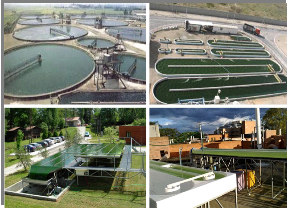
Figure 1. Open pond systems of microalgae cultivation (Acién et al., 2017; El-Baz & Baky, 2018; Narala et al., 2016).
