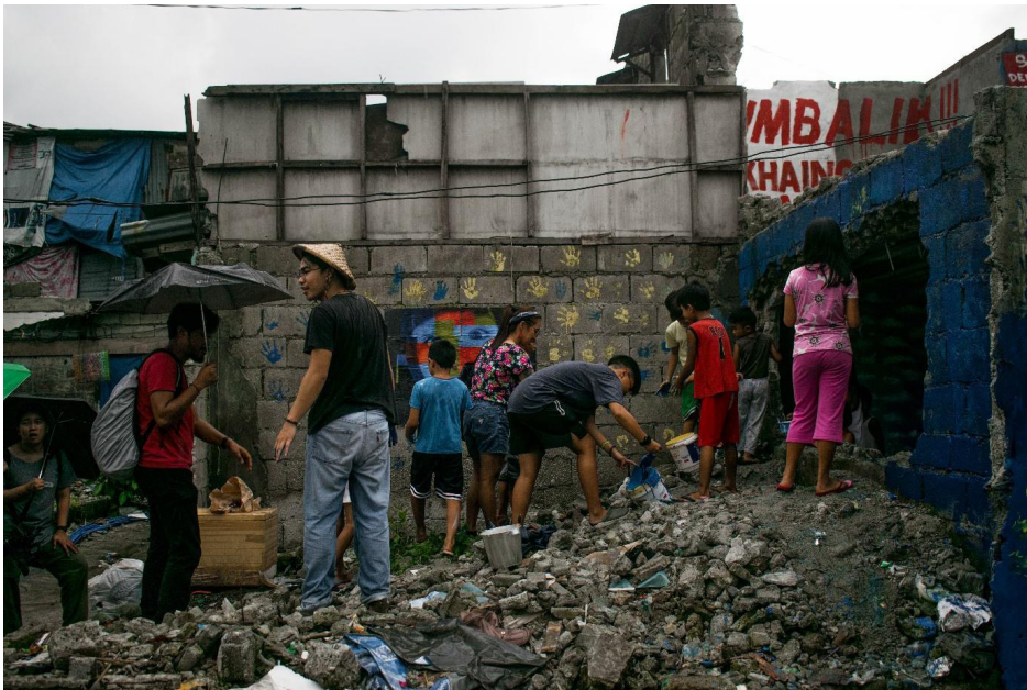
Fig. 1. Locals, including children, and volunteers join to paint handprints on the walls, leaving their mark on a house soon to be demolished. Artmaking activities such as this usually follow a related talk or workshop. Source: Gamilong (2019), permission granted to author.
