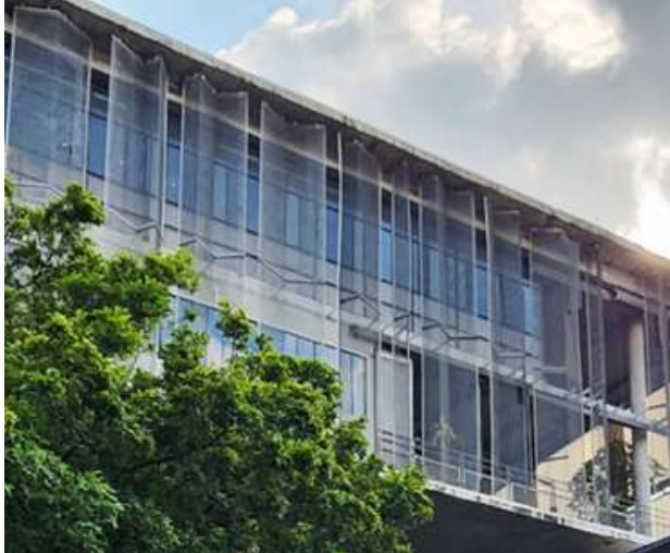
Figure 47. Concrete ledge and expanded metal mesh.
