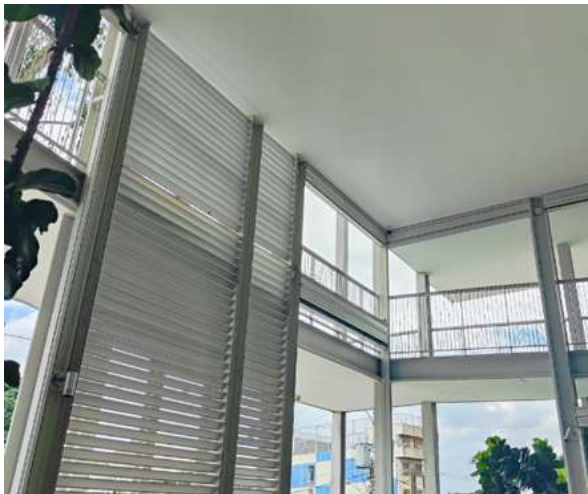
Figure 27. Steel horizontal louvers for shading.
