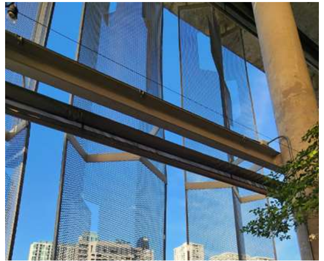
Figure 49. Expanded metal mesh for shading.
