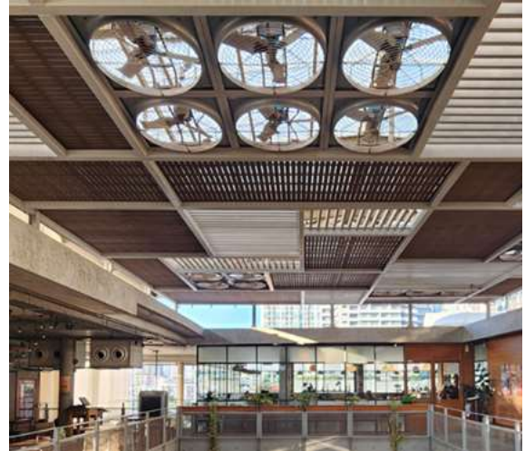
Figure 44. Mechanical ventilation system at the roof. Source: Authors
