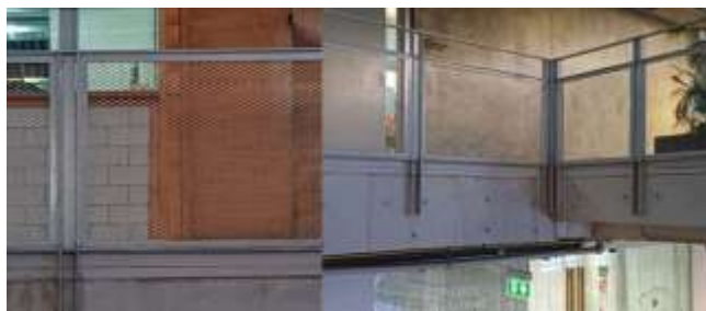
Figure 20. Photo of the expanded metal and railing
