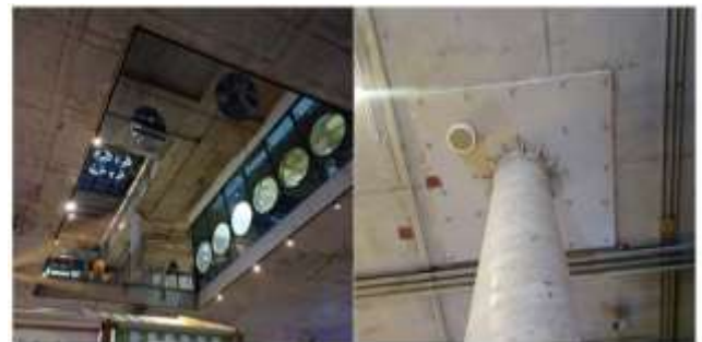
Figure 14. Photos showing the concrete ceiling and the column connection used.
