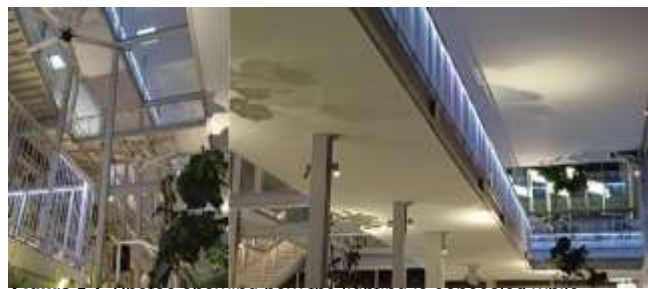
Figure 17. Photos showing how the lighting is concealed while illuminating the railings
