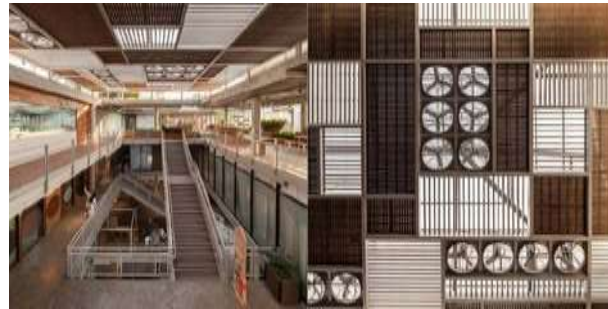
Figure 6. (left) Photo of the third and fourth floor (right) Photo of the ceiling featuring louvers and industrial fans illuminated by a skylight
