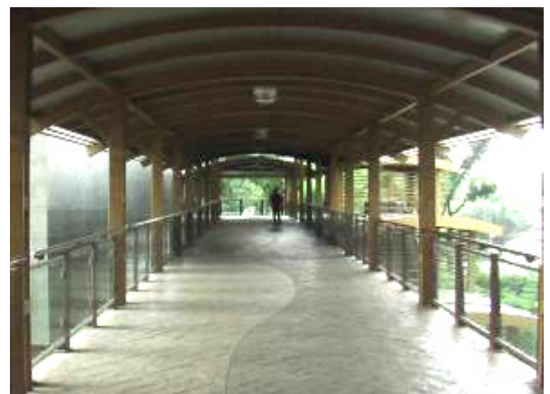
Figure 5: Elevated walkway near Cojuangco Bldg area
