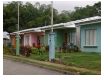
Camino Real Project in rural area
