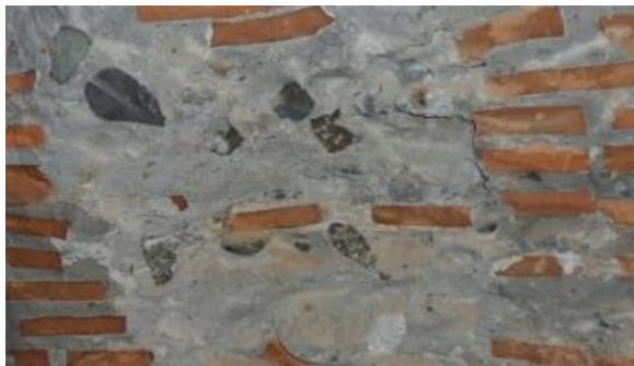
Figure 22. Photo of Brick Wall.
