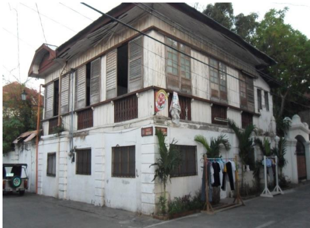
Figure 13. Façade view of Singson House along Mabini Street.
