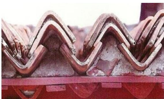
Figure 19. Photo of Clay Tile Roof with Plywood Ceiling.
