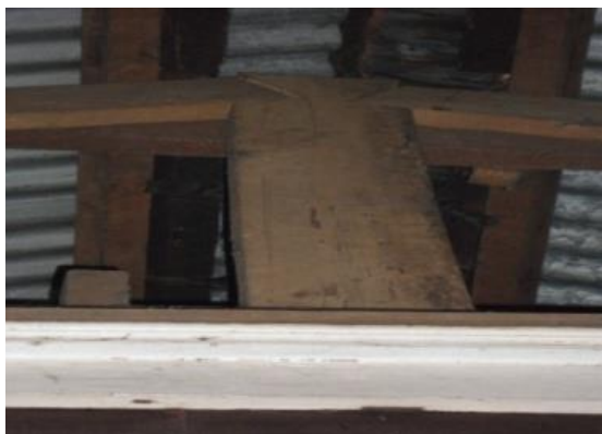
Figure 18. Photo of Metal Roof.
