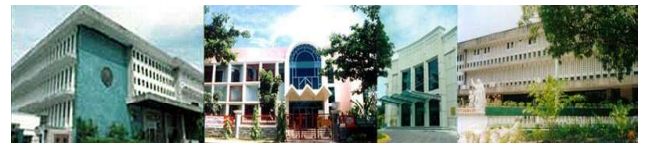
Figure 5 - Upper Grade / Admin (left side), Lower Grade / Performing Arts (middle) Upper Grade / Admin (right side)
