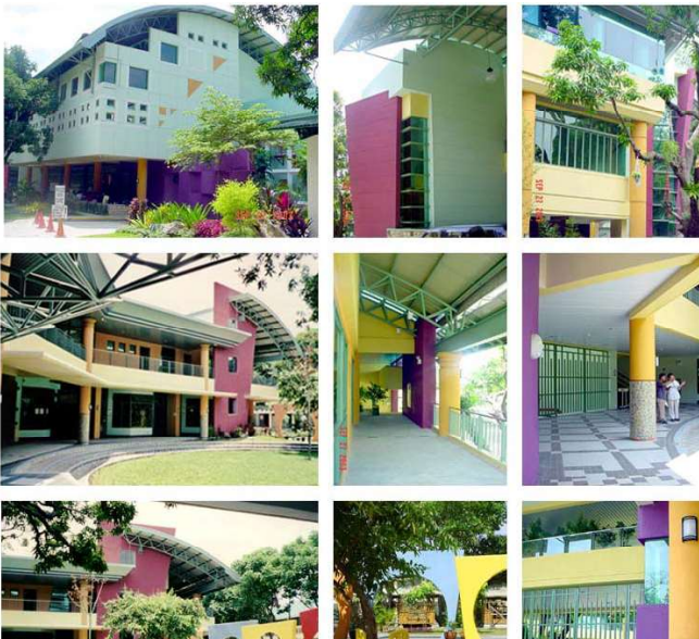
Figure 13 – Buildings on integral development
