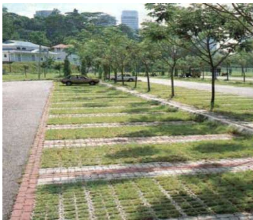
Figure 13 - Grass pavers as an alternative to asphalt parking
