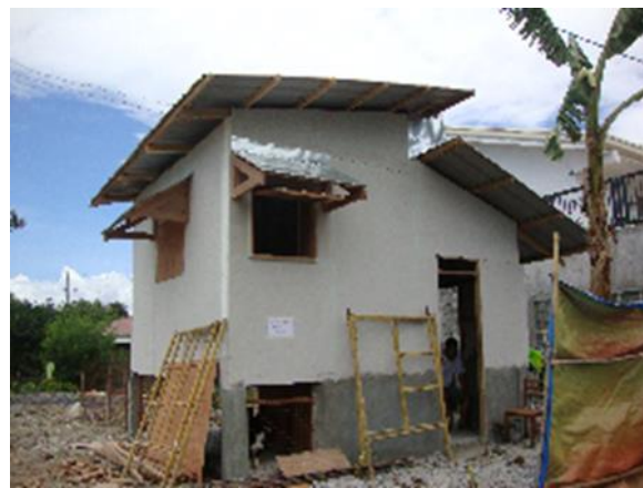
Figure 3. Exterior images of the site.
