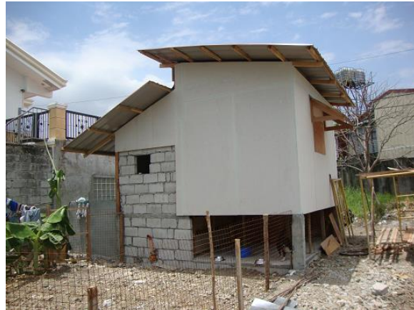
Figure 2. Exterior images of the site: rear view
