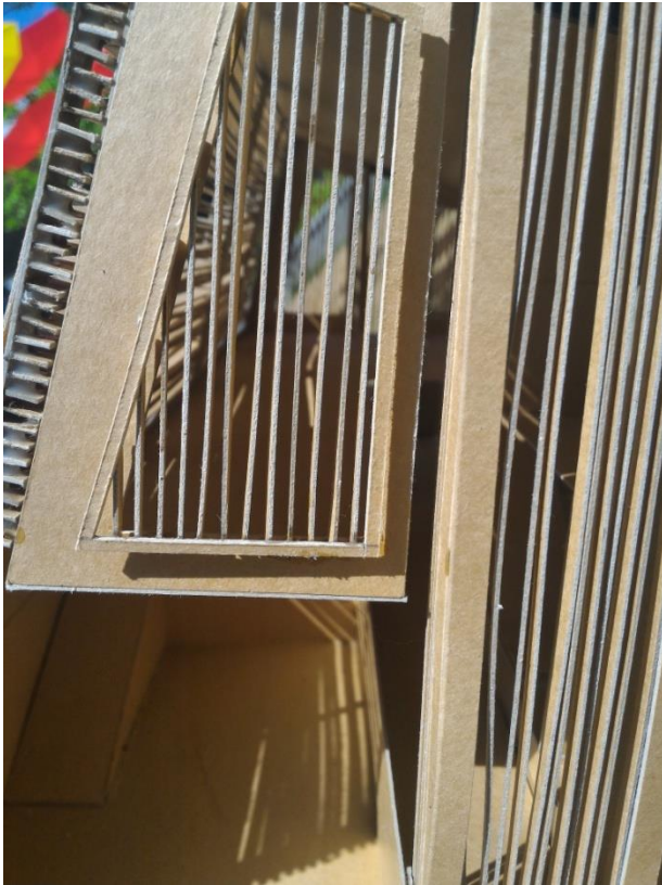
Figure 14: Close up of vertical louvers. Source: Project and photo c/o Kirby Manuel and Kyle Chua (submitted student work)
