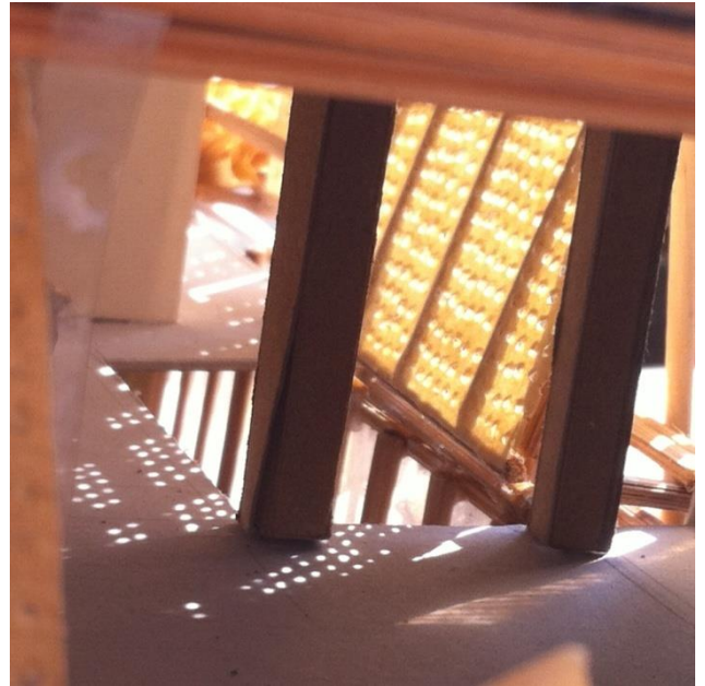
Figure 16: Exterior hallways protected by perforate screens Source: Project and photo c/o Carlo Llanto and Rafael Rulloda (submitted student work)
