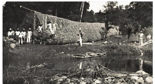
Figure 9. The "Sausage" A Novel method for preventing river overflow on the Tumaga River.
