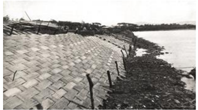
Figure 8. Temporary Bank Revetment, Magat River Control, Bayombong Nueva Ecija.
