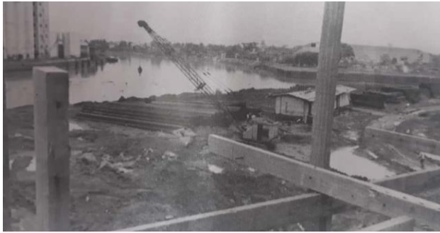
Figure 12. Napindan Hydraulic Control.
