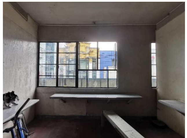
Figure 6. East-facing Window Inlet in Unused Classroom
