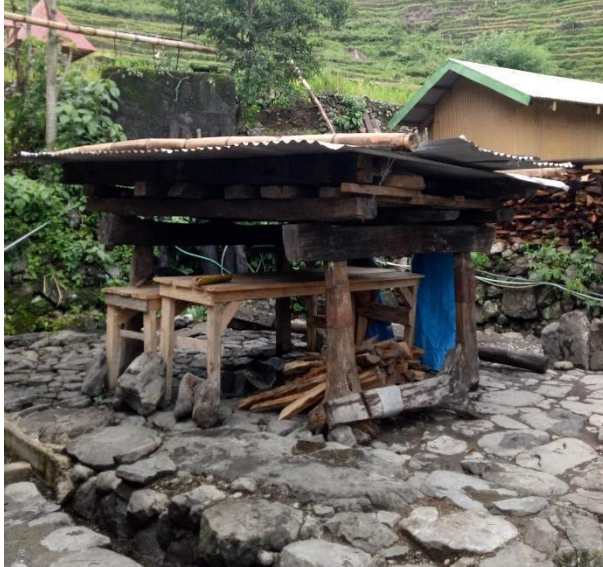
Figure 18. Example of Mode E – Dismantled bale serving as property marker found in Sitio Babloy
