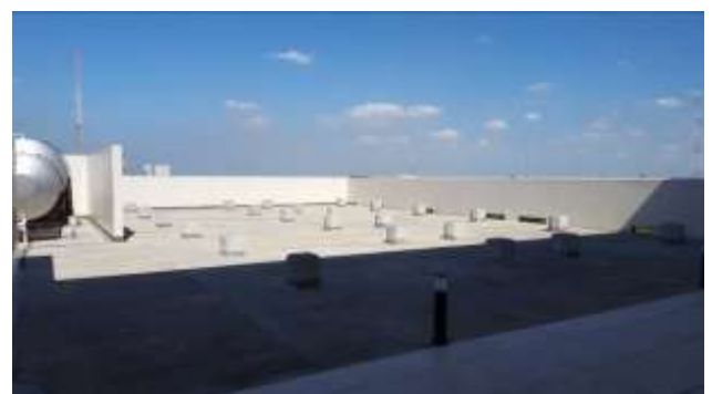
Figure 8. View of a portion of the roof deck area of the UPCA Studio Laboratory Building showing the pedestals for solar panels and water storage tanks.
