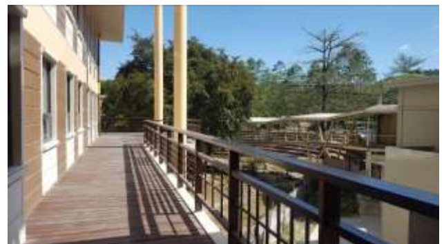
Figure 7. View from the rear balcony of the Studio Laboratory Building of the Bridge connecting UPCA Buildings 1 and 2.
