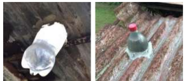
Figure 3. Typical installation viewed from interior (left photo) and exterior (right photo).
