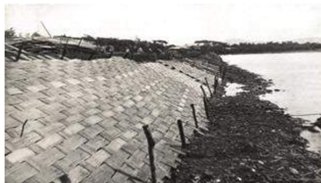
Figure 8. Temporary Bank Revetment, Magat River Control, Bayombong Nueva Ecija.
