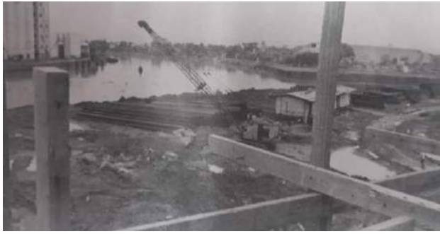
Figure 12. Napindan Hydraulic Control.
