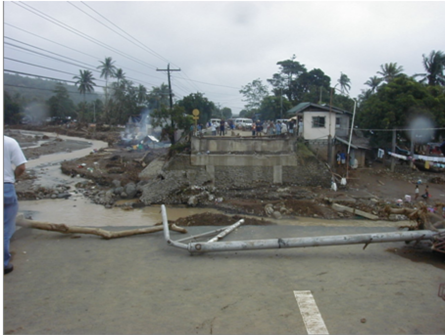
Figure 3. Real Bridge washed out by the flash floods and debris flows (Photo by E. Billedo)
