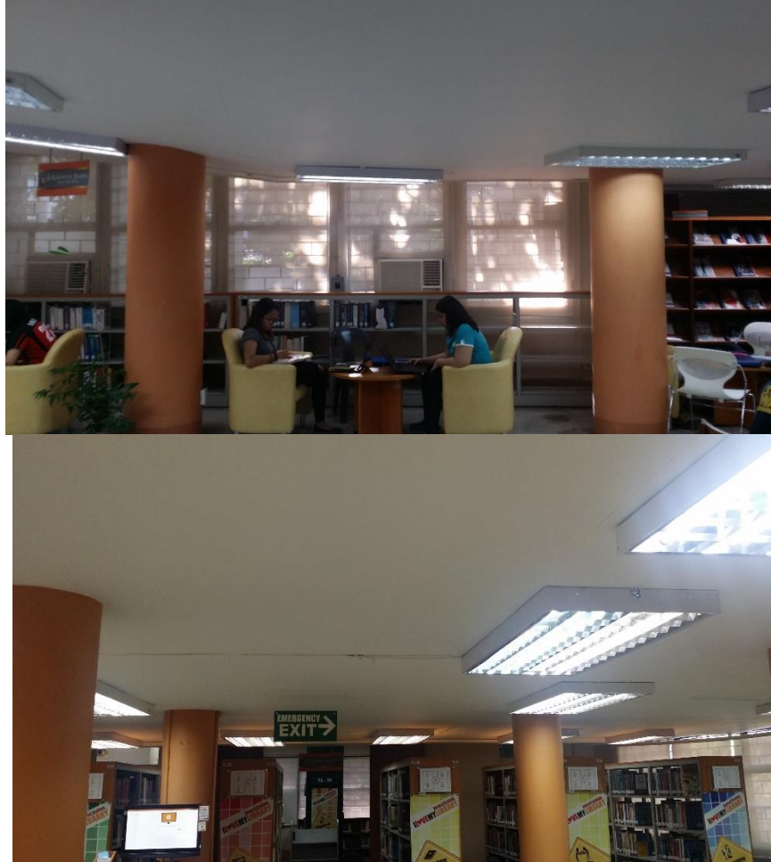
Figure 4. Lighting fixtures placement over tables and shelves at the UPD College of Engineering Library 1
