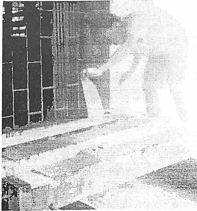
Figure 7. The paper cover is peeled off after the sheet is laid pat
