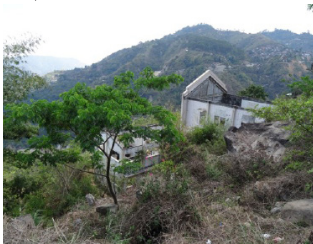
Figure 4: Structures destroyed by a landslide
