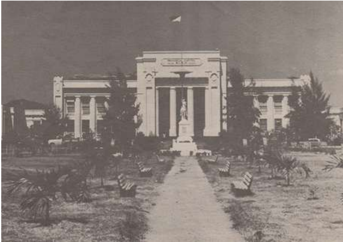
Figure 1. The Capitol building of the Province of Bulacan in the town of Malolos, erected in 1930. Archival photo from Meralco Magazine, April 1958. Courtesy of the Tantoco Family Library and Archives. https://www.flickr.com/photos/28098727@N00/7041932061/in/photostream/
