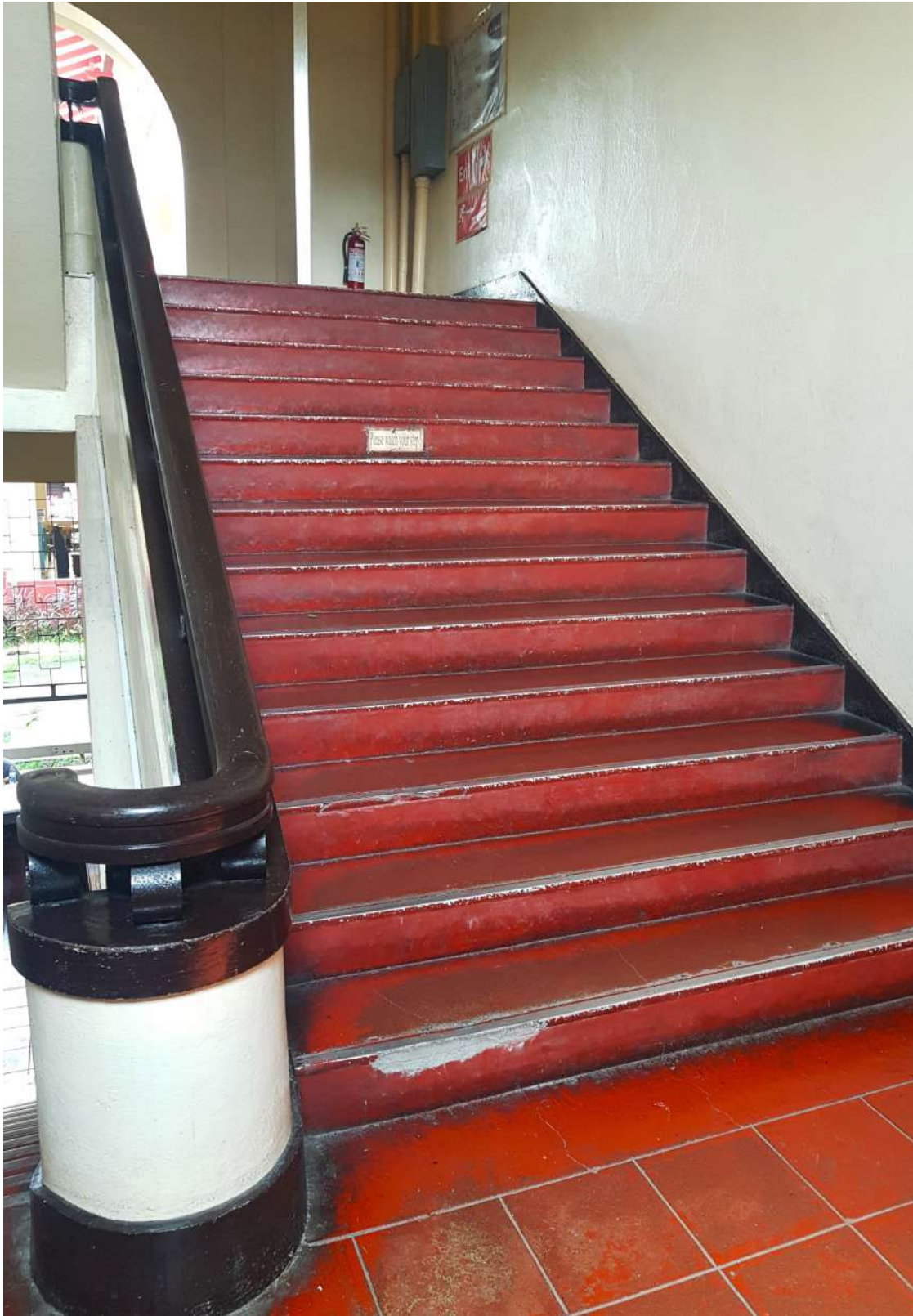
Figure 10. The Benitez Hall's right wing staircase (2022). Source: Author's own.
