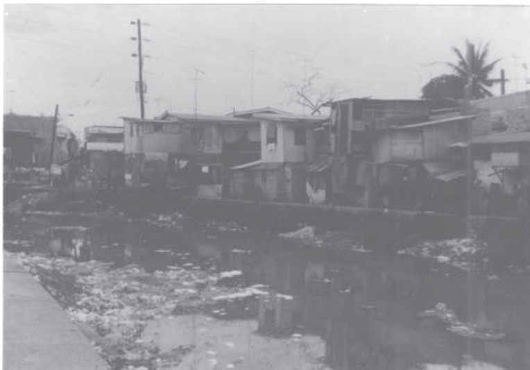
Figure 2. As squatter communities encroach on the drainage canals' service roads, the esteros become inaccessible for dredging activities and solid wastes accumulate on the waterways.
